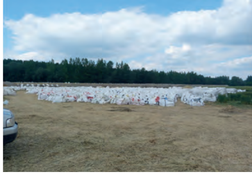
Figure 19. Application of 1 m 3 volume container bag (photo archive of NYUDUVIZIG)
