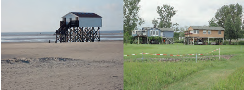
Figure 15. Left: Elevated restaurant at St. Peter-Ording at the North Sea coast. Right: elevated houses near the river Elbe (photos taken by the author)
