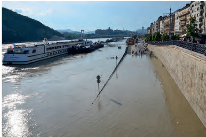
Figure 14. Flood wall in Budapest, Hungary 5
