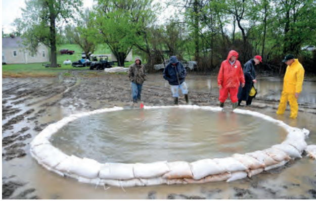
Figure 18. Sand boil created by high exit gradient (sandbags have been piled around the opening to increase the downstream head and reduce the gradient) [10]
