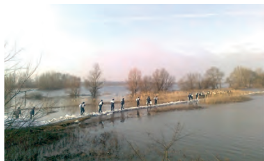
Figure 21. The single line arrival of sandbags during the flood in 2013 on river Marcal (photo archive of NYUDUVIZIG)
