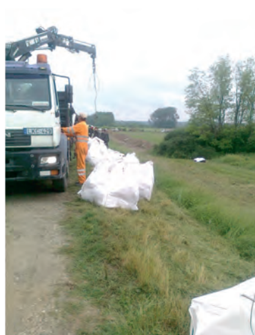
Figure 23. Protective material transport on the dyke (photo archive of NYUDUVIZIG)
