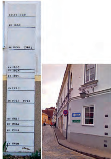
Figure 26. The Danube flood marks, Spitz (Left photo taken from the internet, right photo taken by Pavol Miklánek, 2014)
