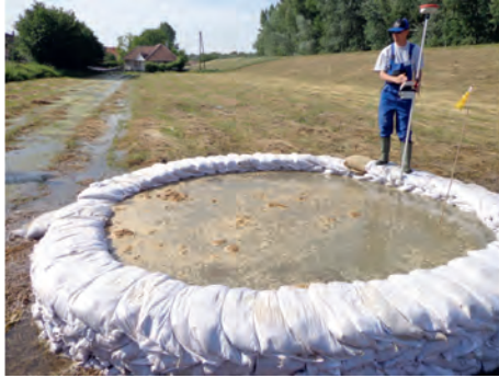
Figure 15. Controlling the built protection structure (photo archive of NYUDUVIZIG)
