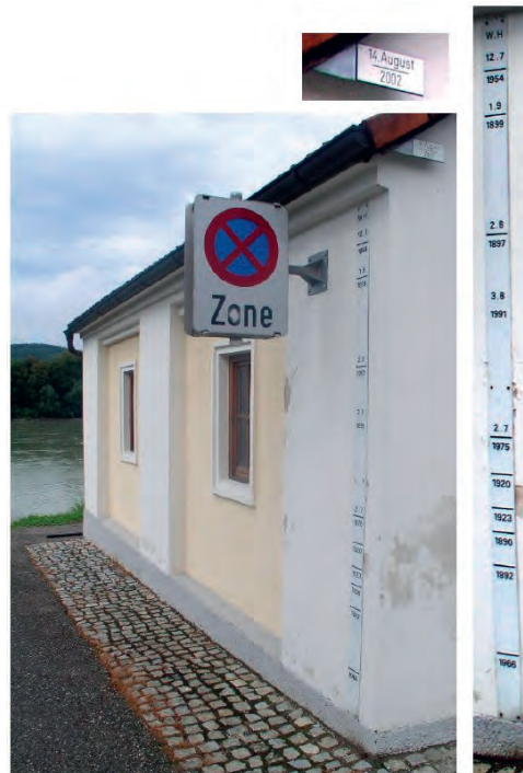
Figure 22. Building with the Danube flood marks in Schönbühel (Photo taken by Pavla Pekárová, 2010.)
