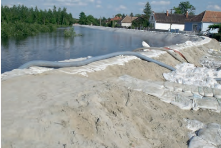
Figure 35. Excess water control without transport possibility on the dike during the flood in 2013 (photo archive of NYUDUVIZIG)
