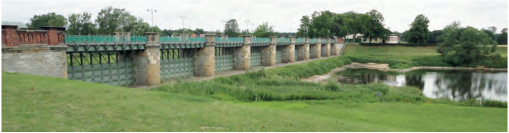
Figure 10. Inflow structure “Pretziener Wehr”, controlling the inflow discharge to the flood relief channel near Magdeburg, Germany (photo taken by the author)
