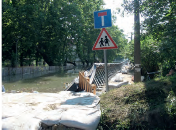
Figure 22. Steel structure based flood barrier, Budapest, 2013 (Budapest Sewage Works Ltd.)
