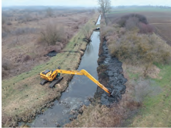
Figure 33. Clearing the drainage canal (photo archive of NYUDUVIZIG)
