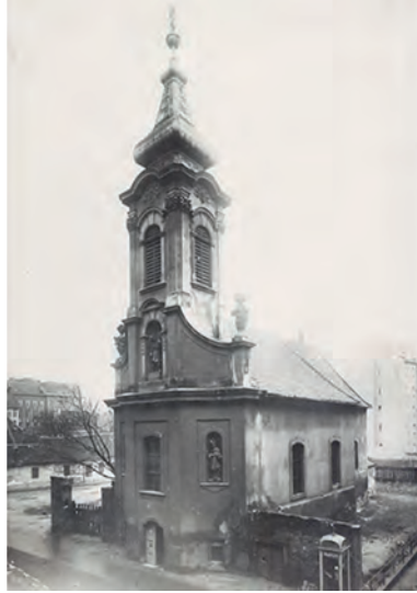
Figure 11. St. Florian Church before its lifting of 1 m in 1937 – the street was raised 60–80 cm after the devastating floods of 1838 and 1876 [15]
