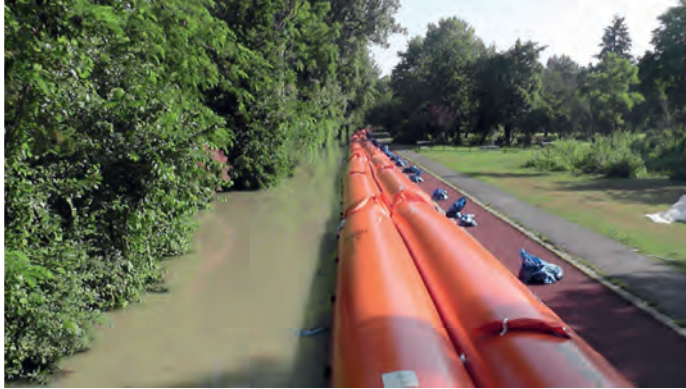
Figure 21. Inflatable barrier during the 2013 Budapest flood (Budapest Sewage Works Ltd.)
