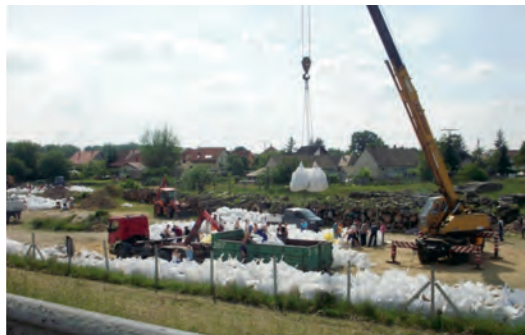
Figure 20. Sandbag filling in a central filling station of Győr during the flood in 2013 (photo archive of NYUDUVIZIG)
