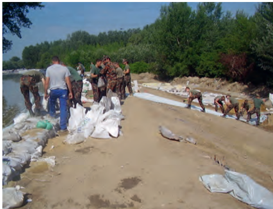
Figure 24. The sandbag slides on foil down the slope (photo archive of NYUDUVIZIG)
