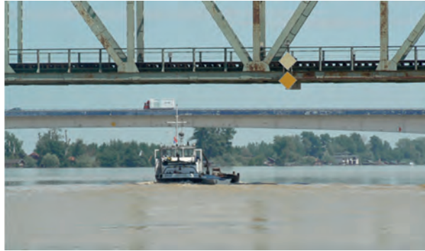
Figure 17. Navigation under the Belgrade bridges during floods, 2014 [30]
