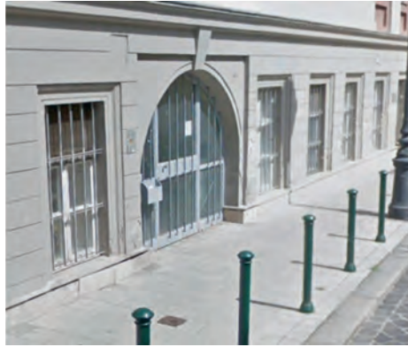
Figure 9. Raised street section in Budapest – Veres Pélné street (Google street view)
