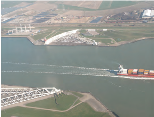
Figure 2. Maasdijk, tide gate at Rotterdam [7]
