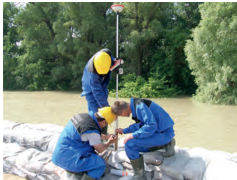
Figure 14. Controlling the height of the levee (photo archive of NYUDUVIZIG)
