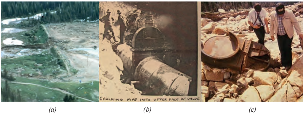
Figure 4. Lawn lake a) embankment after failure; b) gate valve improperly installed; c) recovered gate valve 70 m downstream [14]
