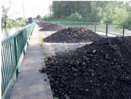
Figure 16. Bridge protection during the flood (photo archive of NYUDUVIZIG)
