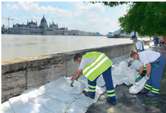
Figure 15. Low flood protection wall as part of a wharf in Budapest – flood control operation in progress in 2013 (Budapest Sewage Works Ltd.)
