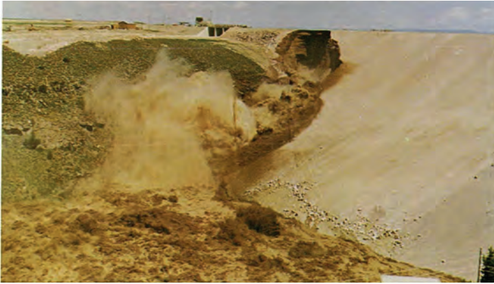
Figure 3. Teton Dam showing progressive piping up to breach [24]
