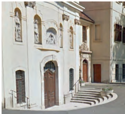
Figure 10. St. Rokus Church in Budapest – raised street level at the entrance of the church (Google street view)
