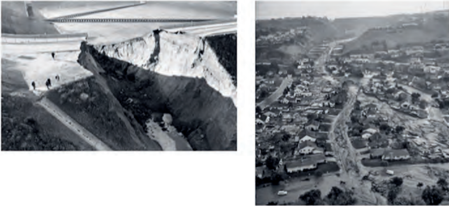
Figure 5. Reservoir flood in Los Angeles, 1963 ( http://damfailures.org/case-study/baldwin-hills-dam/ )
