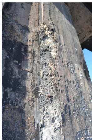
Slope side of the pier
