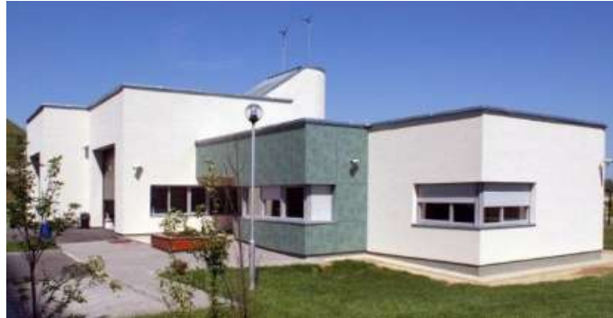
2. Figure. Office building constructed in passive house style [2]
