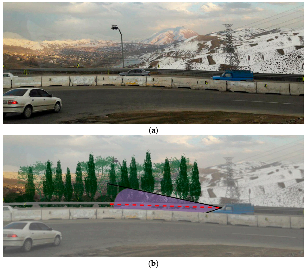
Figure 12. (a) Dangerous bend with distracting views, (b) sight obstruction simulation.
