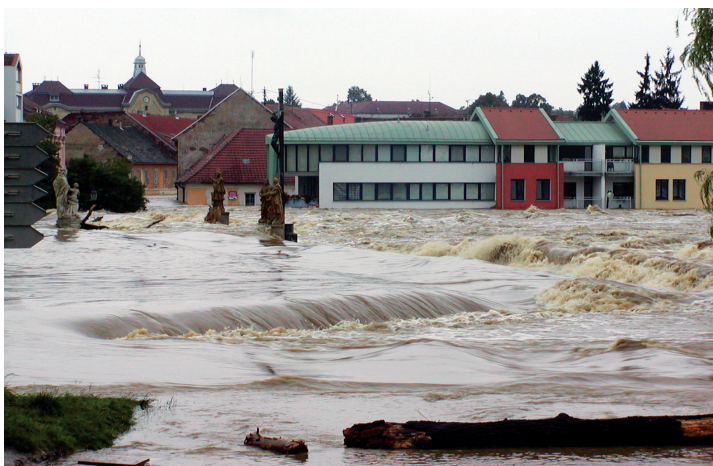
Figure 12. Bridge over the river Písek
