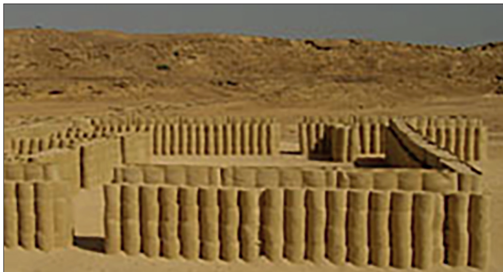
Figure 3: DEFENCELL protective wall 8
