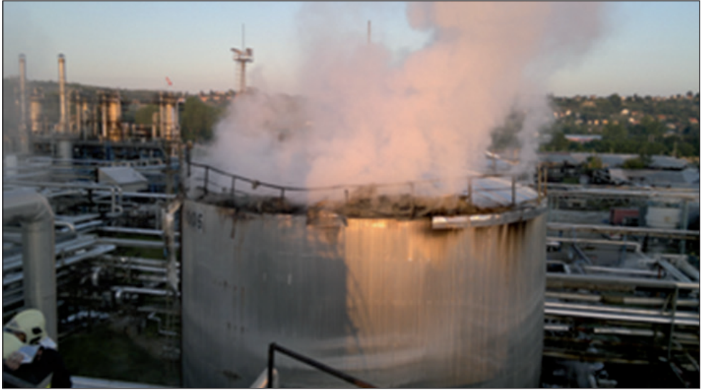
Figure 5: Explosion and fire in bitumen producing factory [14]
