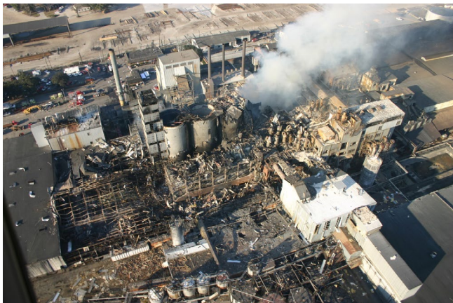
Figure 1. Imperial Sugar Refinery after explosion of sugar dust [4]
