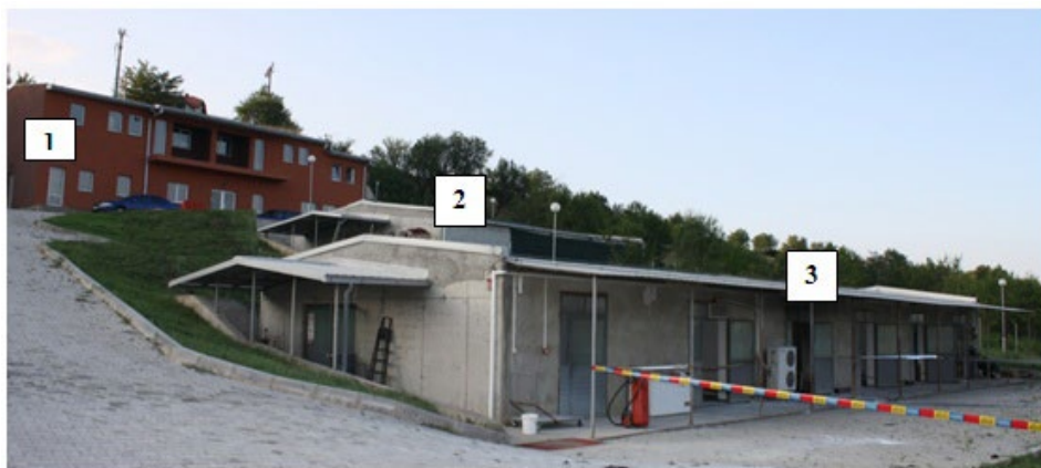
Figure 2. Facility for production pyrotechnical materials
